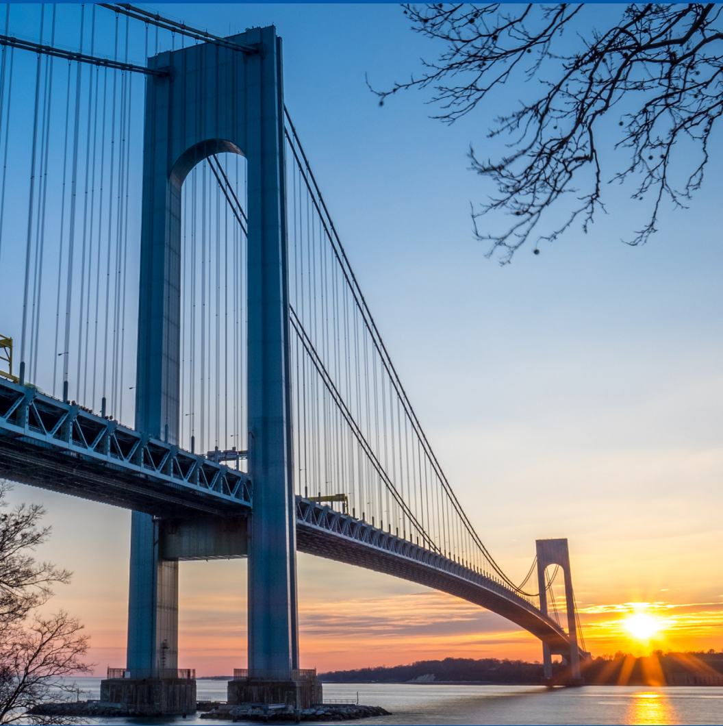
Verrazzano-Narrows Bridge, Staten Island, NY
