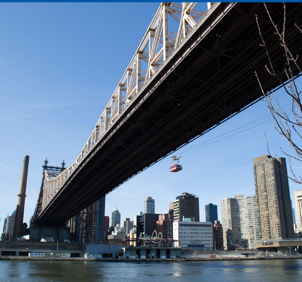
Ed Koch Queensboro Bridge, New York, NY
